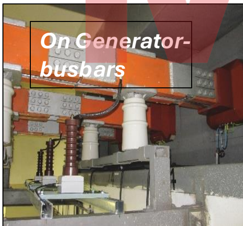
Examples of coupling capacitors installations
