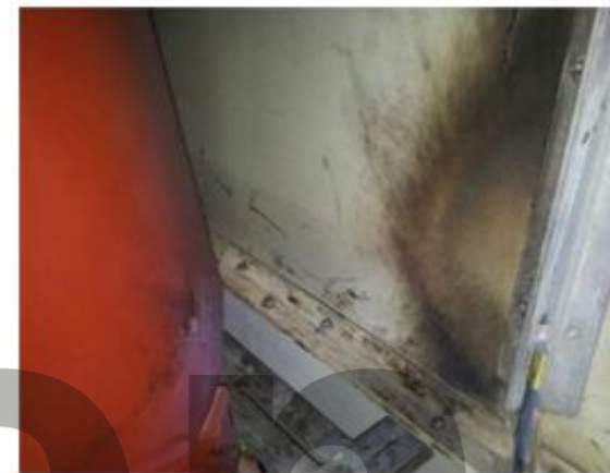
Figure: Flashover in transformer tank wall
